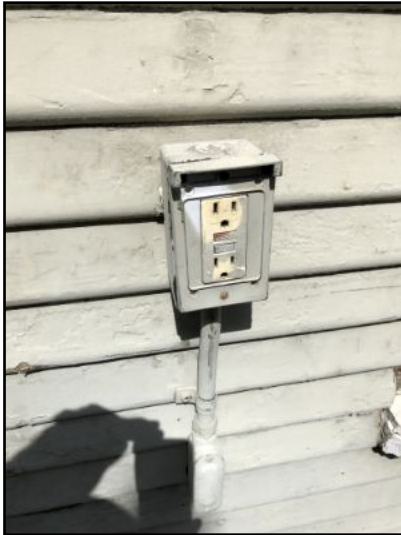
broken weather cover - along the driveway side of home
