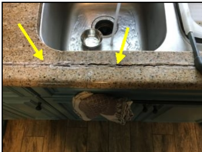
damaged counter top
