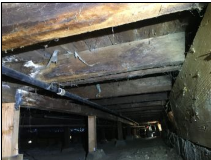
floor joists appear to be in fair condition
