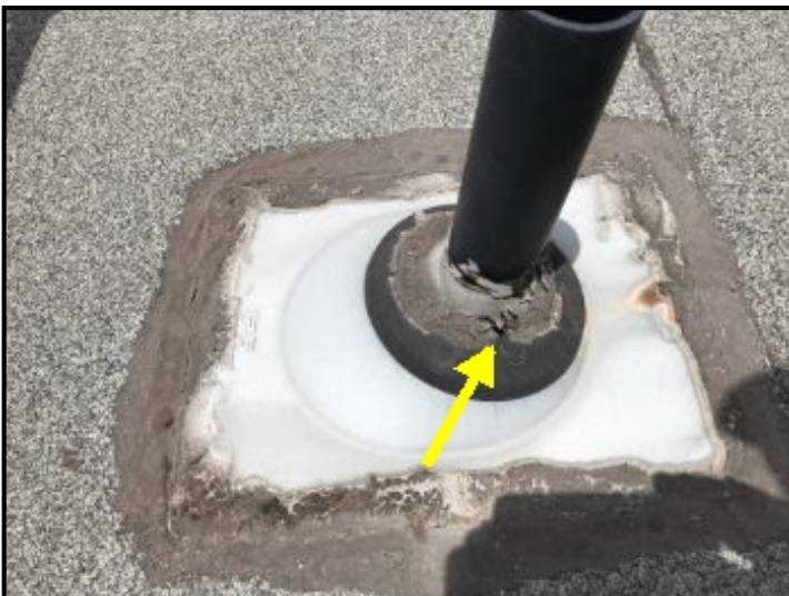
mastic cracking
