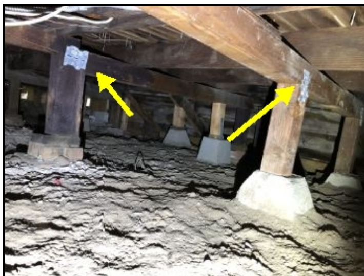
strapping added to posts
