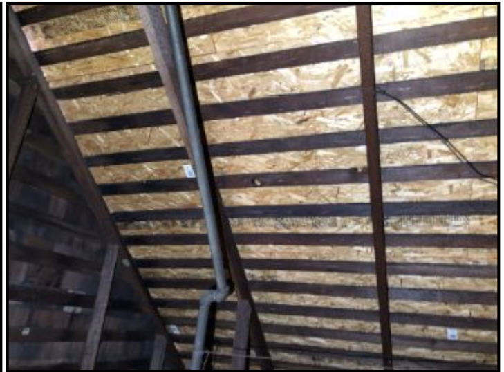
Spaced sheathing with OSB sheathing
