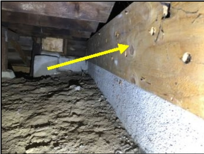
Plywood applied to cripple walls
