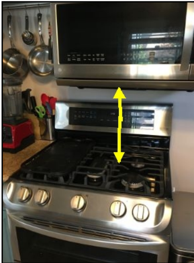
microwave too close to burners
