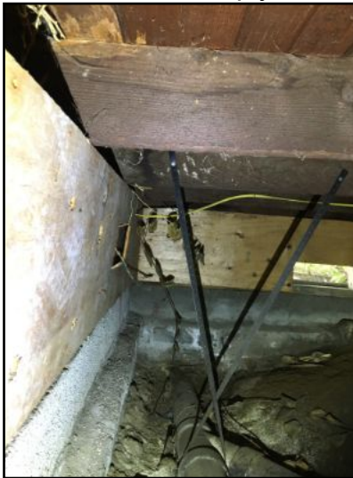
plywood applied at west and north walls
