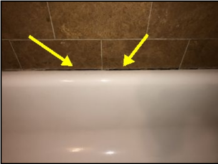
staining f grout
