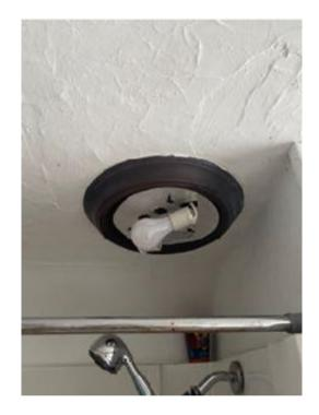
**Q** Monitor The bathroom overhead lighting was not functional. Repairs/replacement recommended
